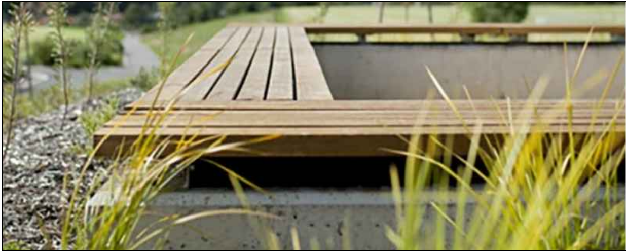
Masonry wall with cantilever timber seating
